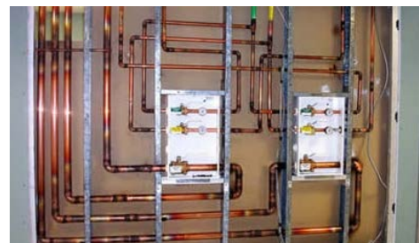
Typical commercial medical gas installation rough-in.
