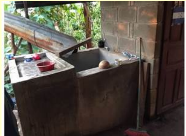
A pila in an area home. This is the kitchen sink, kitchen counter, laundry machine, water storage container, and general washing area for a traditional Honduran home
