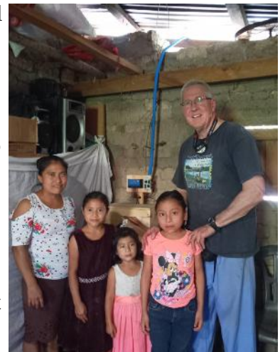
Solar Install Sayli's house completed Jan 2024
