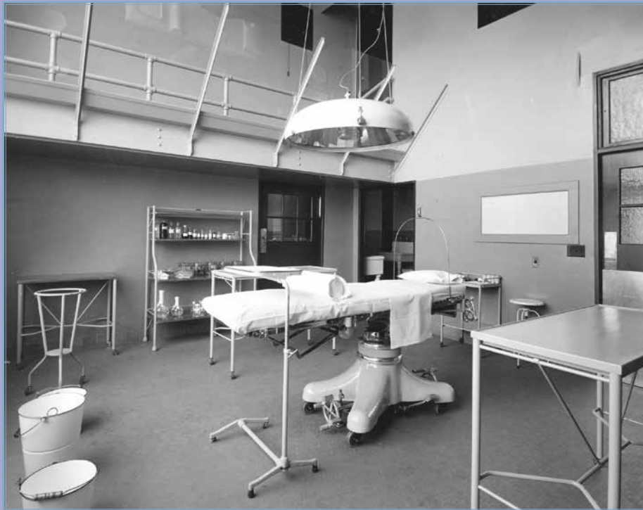
Fifth Floor Operating Room, 1926 (Note viewing balcony).
